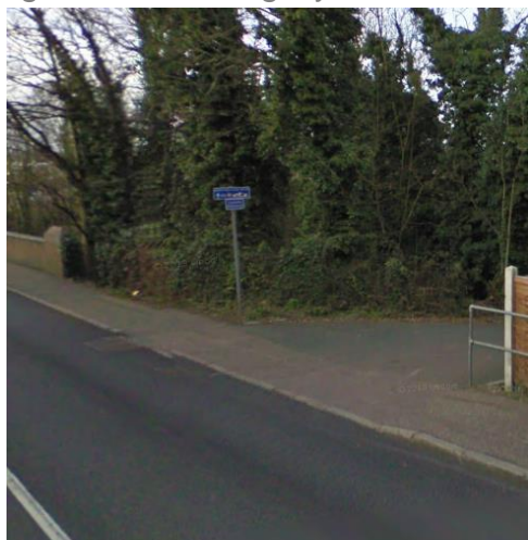
Figure 4.2 Existing Cycle routes ends abruptly at Parkeston Road
